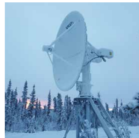
One of our antennas at the Canadian Satellite Ground Station.
